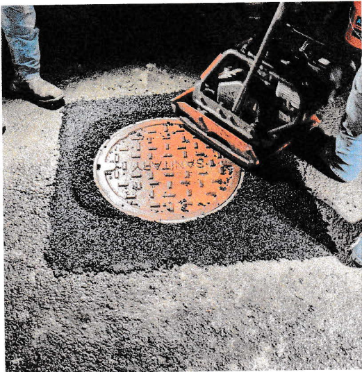
3. Temporary Patch with new cover at grade
