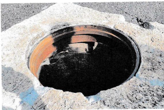
1. Failure – manhole frame sinking in
