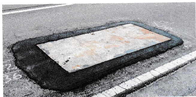
2. Temporary Repair – metal plate and asphalt patch
